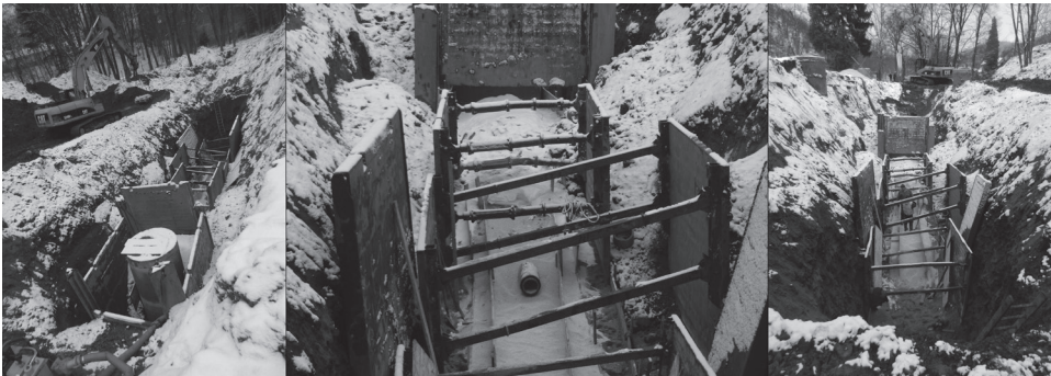
Rys 3. Budowa studni S-1 Fig 3. Building of the S-1 well
